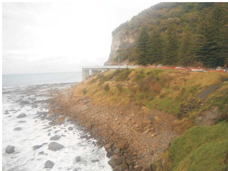
Figure 2 – Northern Amphitheatre embankment erosion following storm event on 6 June 2012 (photograph date 14 June 2012)
